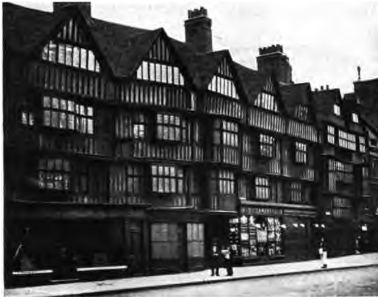
AN ARCHITECTURAL TYPE WHICH HAS FURNISHED MUCH LATTER-DAY INSPIRATION (Old houses in Holborn, London)
